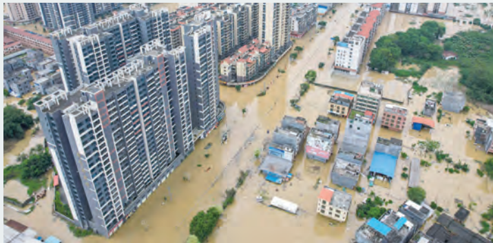
A view of flooded buildings and streets after heavy rains in Qingyuan city, China. – AFP
