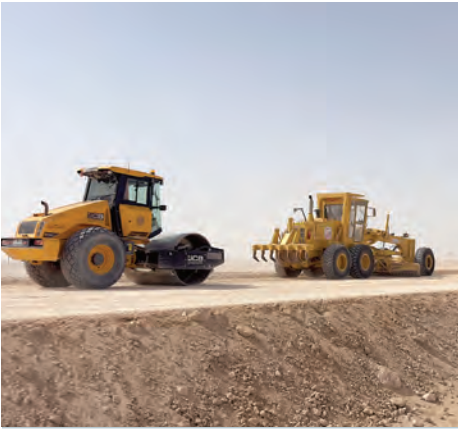
Heavy equipment, construction vehicles, earthmoving works and road preparation activities were visible along various stretches of the route.
