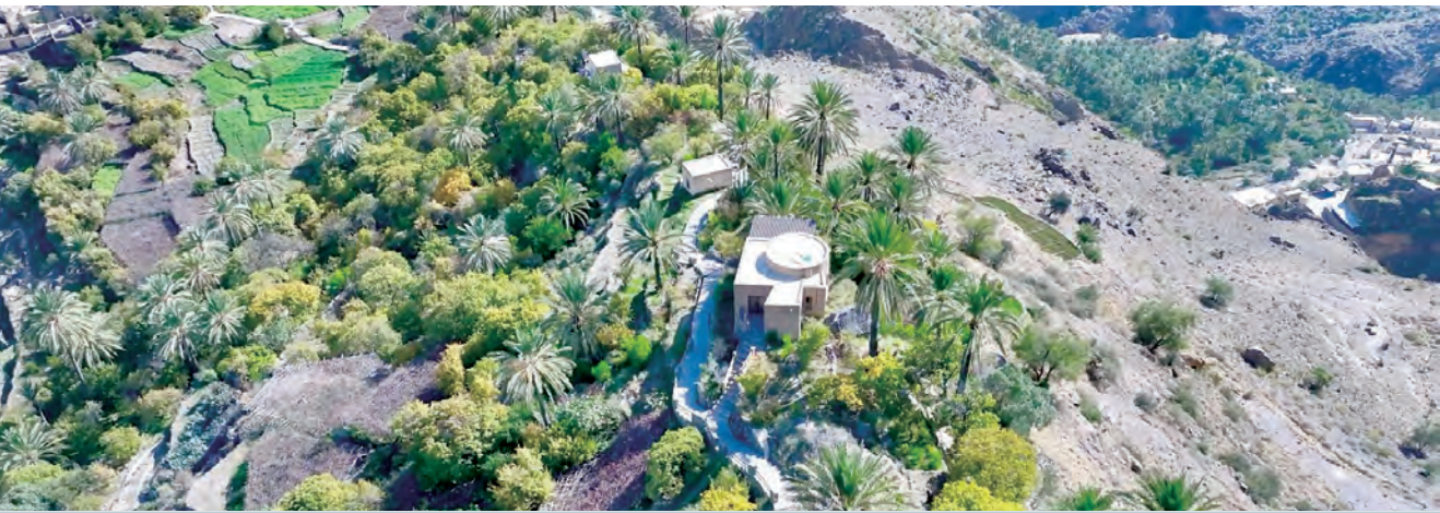
The project includes the construction of a main road with a length of 6.5 km, in addition to a 2.2-kilometre link road.
