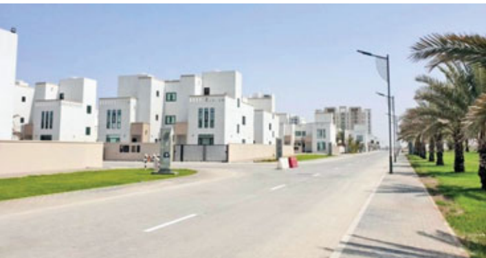
SOROUH PROJECT: Al Naseem Neighbourhood, which constitutes the first project of Sorouh Initiative, comprises 220 housing units.
