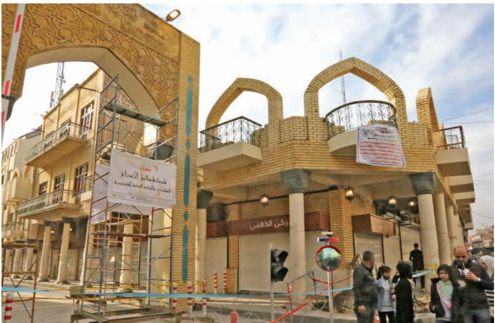
Iraqis walk past the cordoned-off entrance to the landmark street of Al-Mutanabi, which is specialised in book sales and due to reopen soon following extensive renovation, in Baghdad on Friday (AFP)
