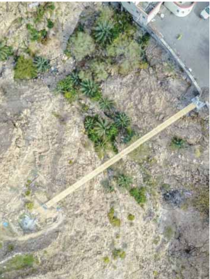
MUHANNA AL ZAIDI from Wadi Fida, Wilayat of Dhank was able to construct a suspension bridge with a length of 40 metres and a height of 13 metres. The lengths of wires used reached one kilometre to ensure the rigidity and cohesion of the bridge to ensure safety measures.
