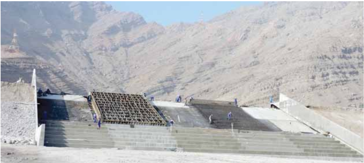
With the aim of supplying water resources and providing protection from flood risks, the government has completed 67 per cent of Wadi Ghumdah in Wilayat of Bukha in Musandam governorate. – ONA
