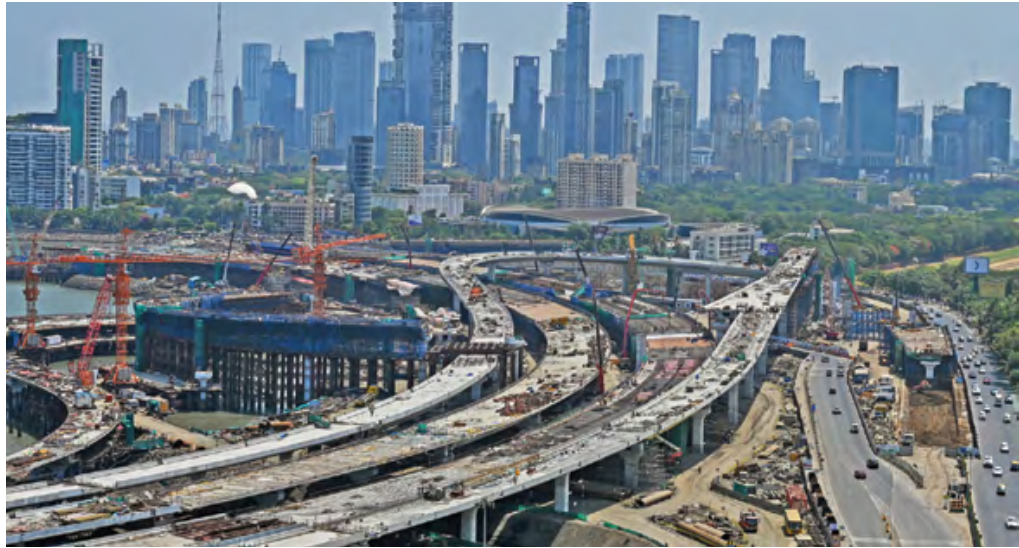
The city skyline is seen beside a construction site of a coastal road project near Haji Ali mosque in Mumbai on Wednesday (AFP)
