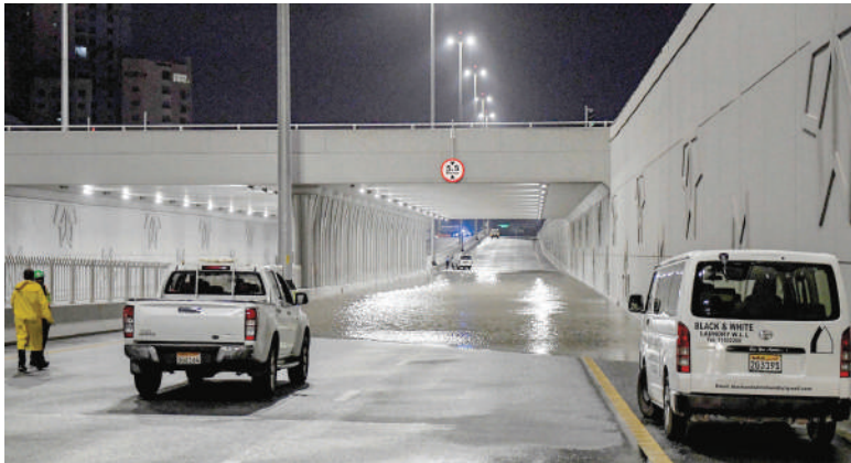
Road workers and rescue crew close a section of Al-Fateh Highway in Bahrain's capital Manama after rainwater flooded it on Tuesday. — AFP
