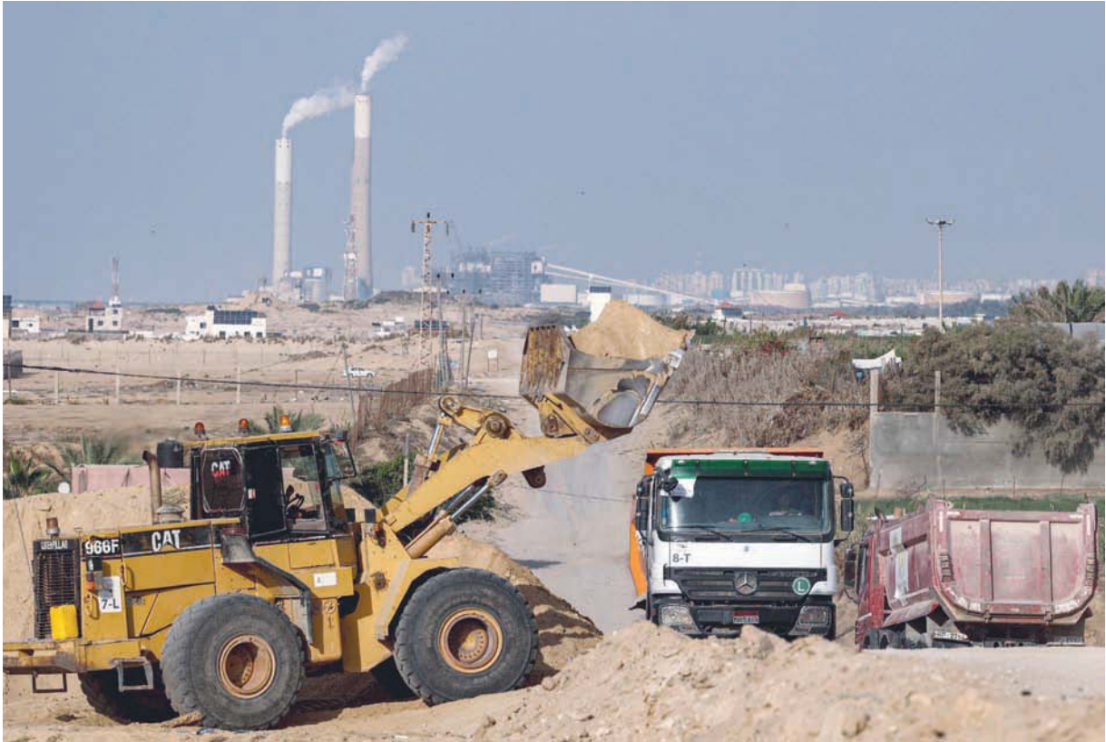
An excavator clears land at a road section undergoing expansion north of Gaza City. — AFP
