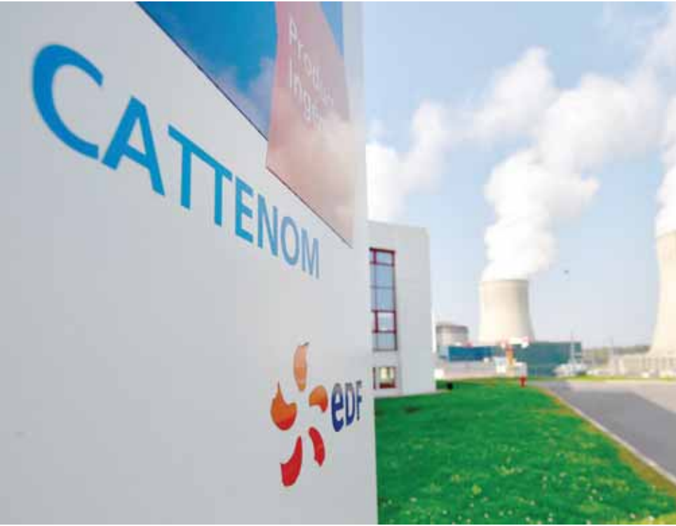
The cooling towers of the nuclear power plant at Cattenom in eastern France. French energy giant EDF (Electricite de France) announced on August 24 it was prolonging the shutdown of four nuclear reactors due to corrosion risks, amid rising energy prices. – AFP
