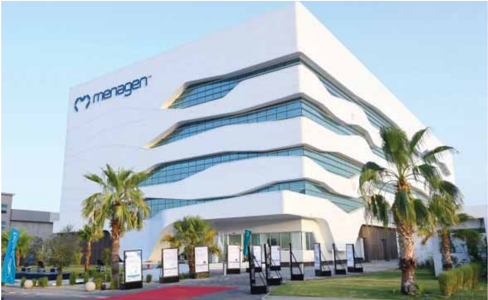
The Menagen Pharmaceutical Industries Plant
