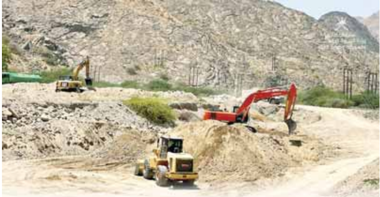
Construction under way on Wadi Adai dam.
