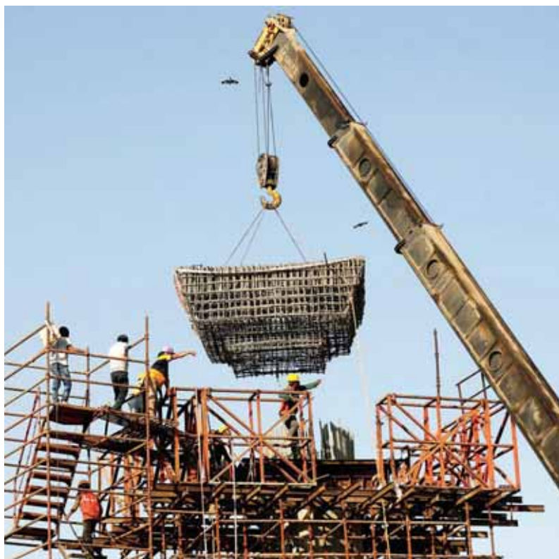
Workers build a pillar at the site of the metro railway flyover under construction in Ahmedabad, India. — Reuters
