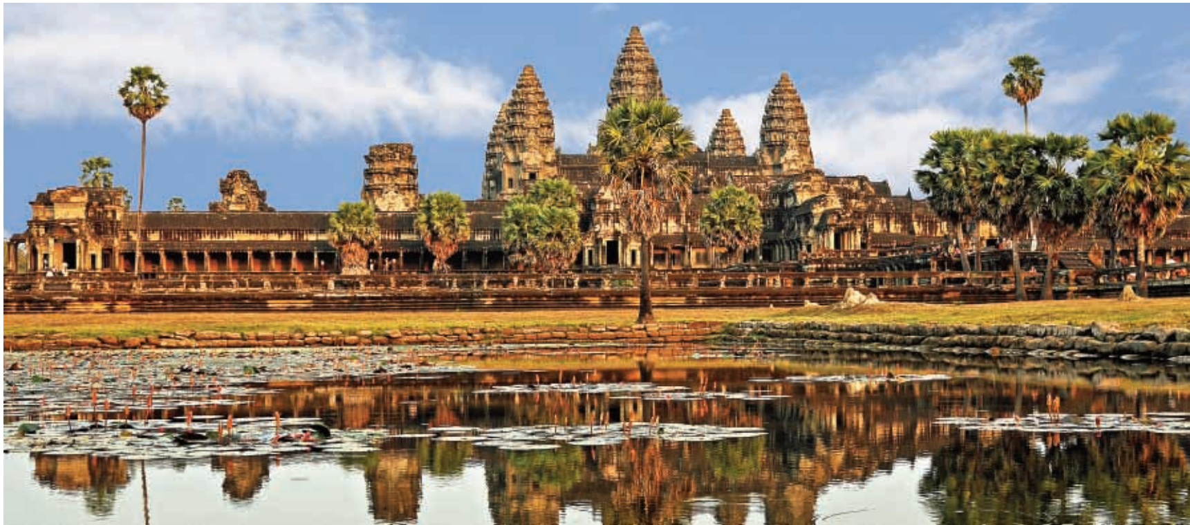
The conservation of the 12 th century Angkor Wat temples between 1986 and 1992 is perhaps the most outstanding project that the ASI has undertaken outside India
