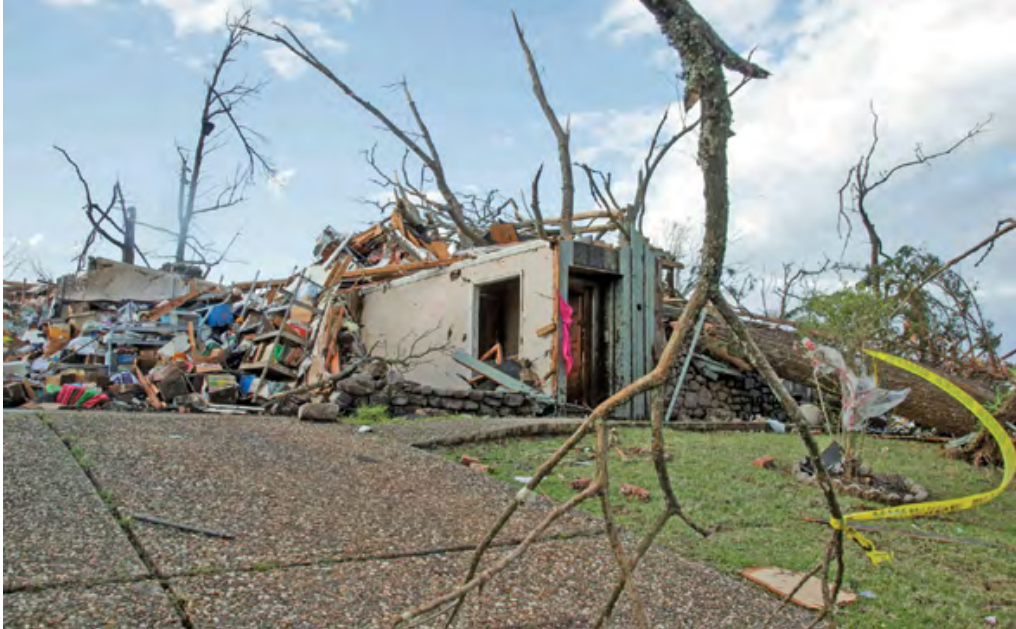
Homes damaged by a tornado are seen on Friday in Little Rock, Arkansas (AFP)
