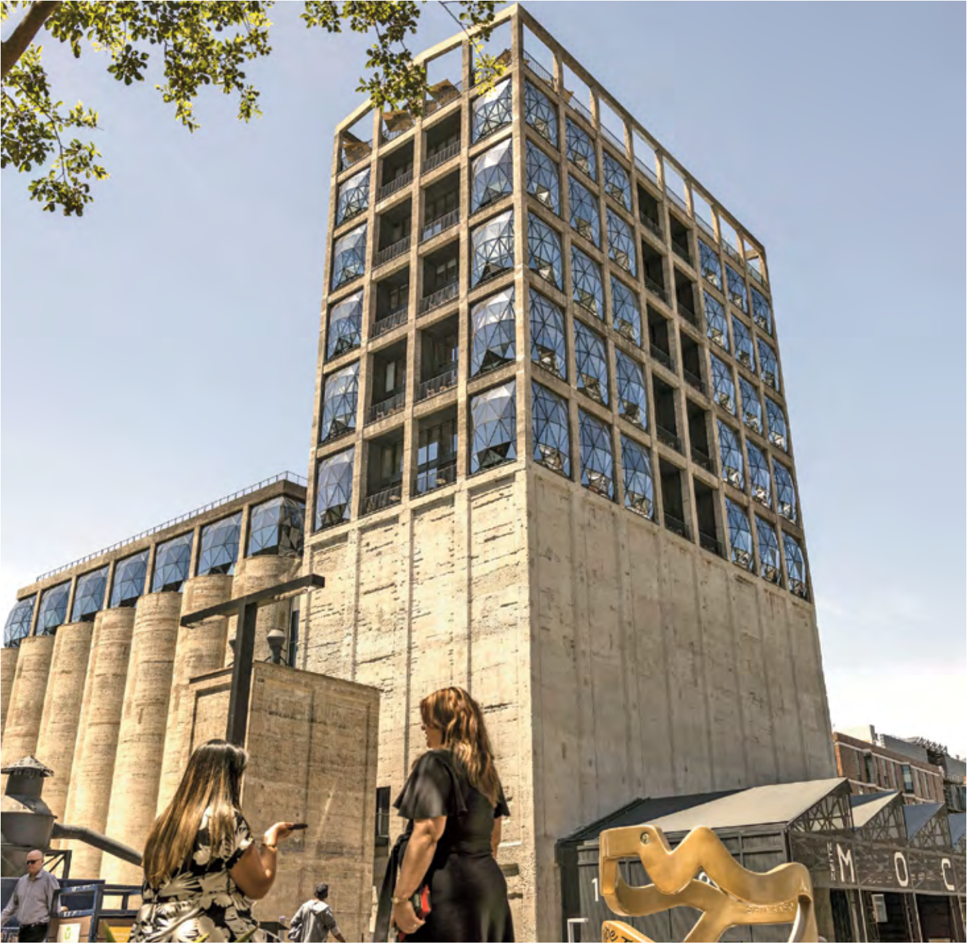
A general view of the Zeitz Museum of Contemporary Art Africa (MOCAA) in Cape Town
