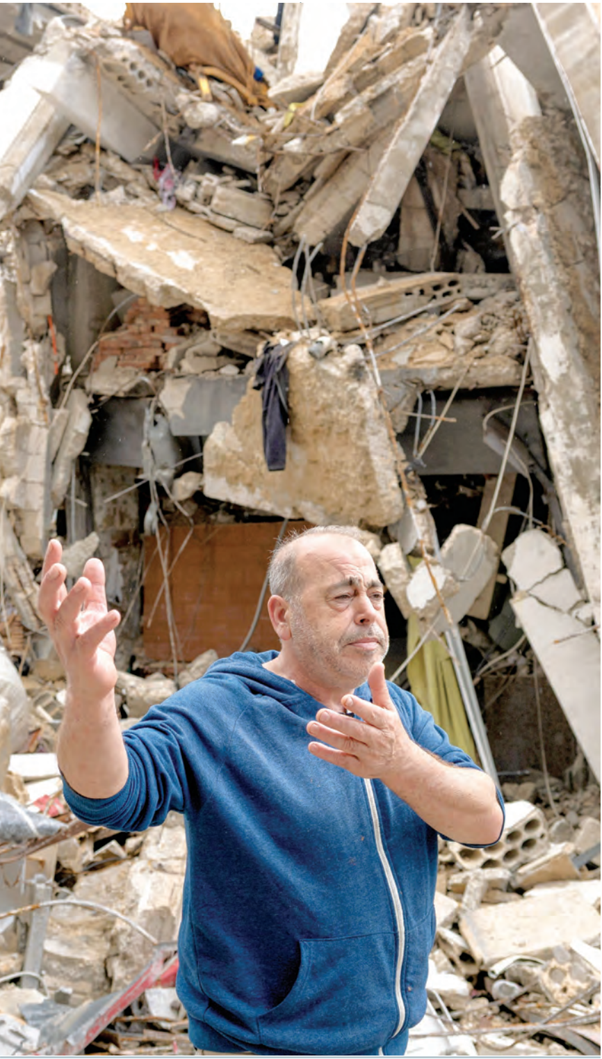
A man gestures as he stands in front of a building damaged in an Israeli strike in Tyre, Lebanon, on Sunday. — Reuters
