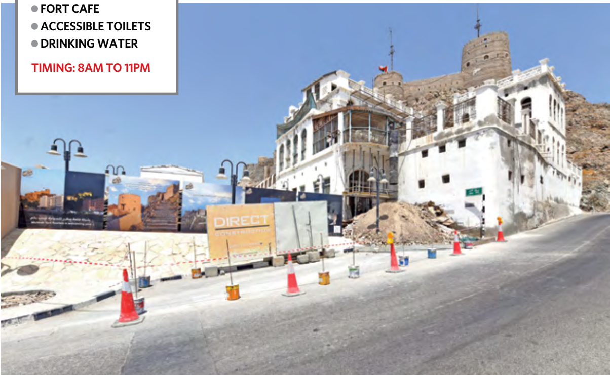
A section of the adjacent road, near the entrance at the rear end of the fort complex, has been cordoned off to facilitate works
