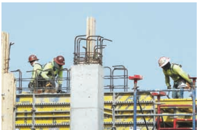
Workers are seen on a construction site in Miami, US on Friday (AFP)
