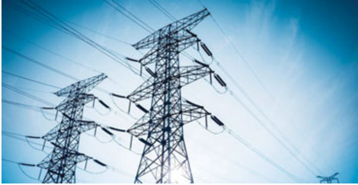
NETWORK CAPACITY: Muscat Electricity Distribution Company has increased its network capacity in the Muscat Governorate by 122 mega-volt-ampere during the first half of 2020. - File picture
