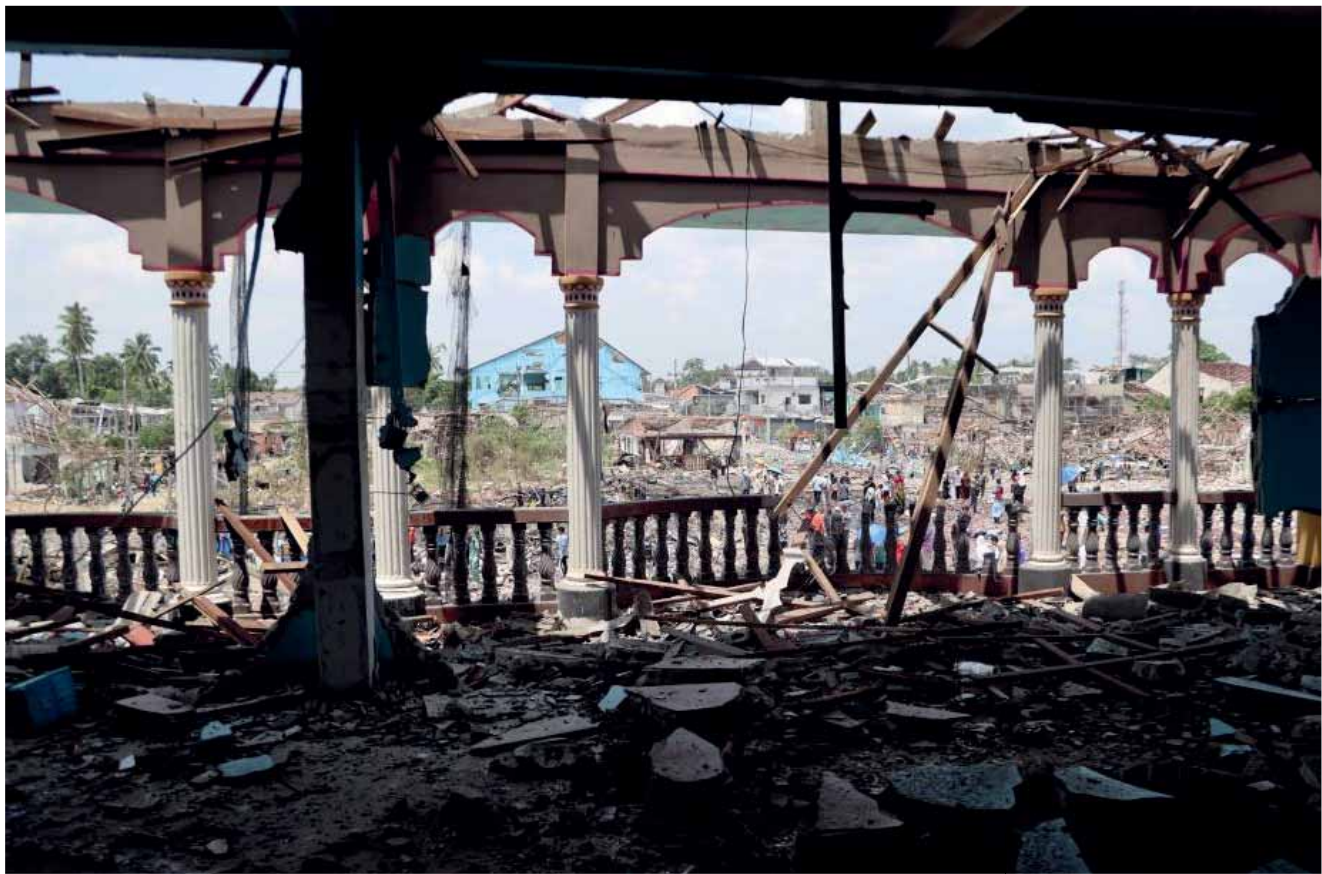
10 killed in fireworks warehouse explosion in southern Thailand This picture shows the scene of explosion in Narathiwat, Thailand. At least 10 people were killed and more than 100 were injured after a fireworks warehouse exploded in southern Thailand on Saturday, government officials said. Xinhua
