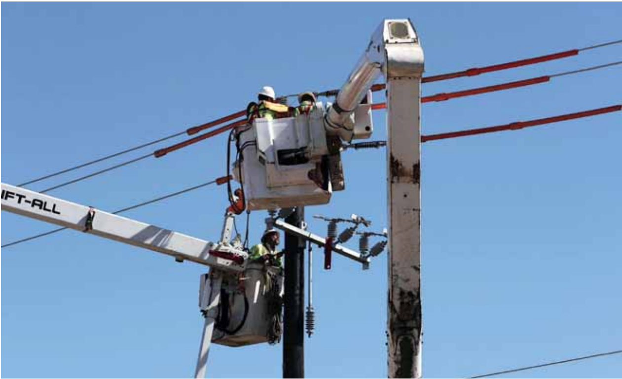
Workers install a utility pole to support power lines after an unprecedented winter storm in Houston, Texas, on Monday. — Reuters
