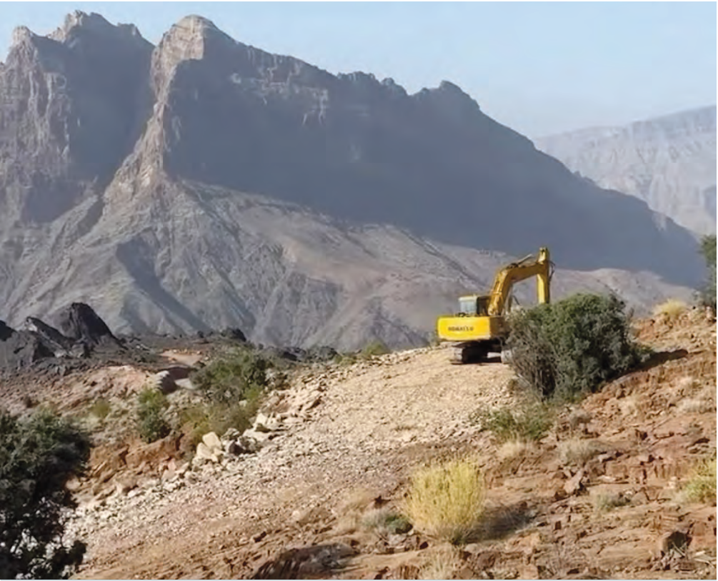
The road is expected to strengthen social ties between residents of Al Awabi and Al Hamra.
