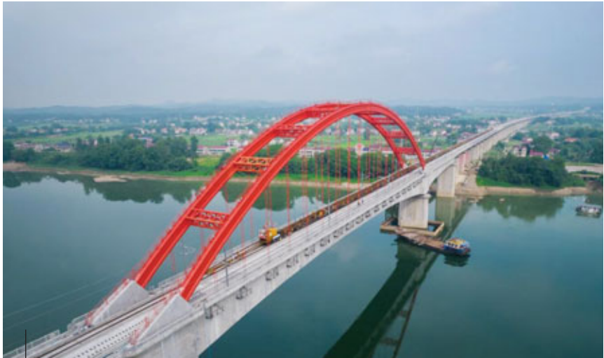
Zishui bridge along Changde-Yiyang-Changsha railway under construction Aerial picture shows a track-delivery vehicle passing through the Zishui super major bridge along Changde-Yiyang-Changsha railway, in central China's Hunan Province. Xinhua
