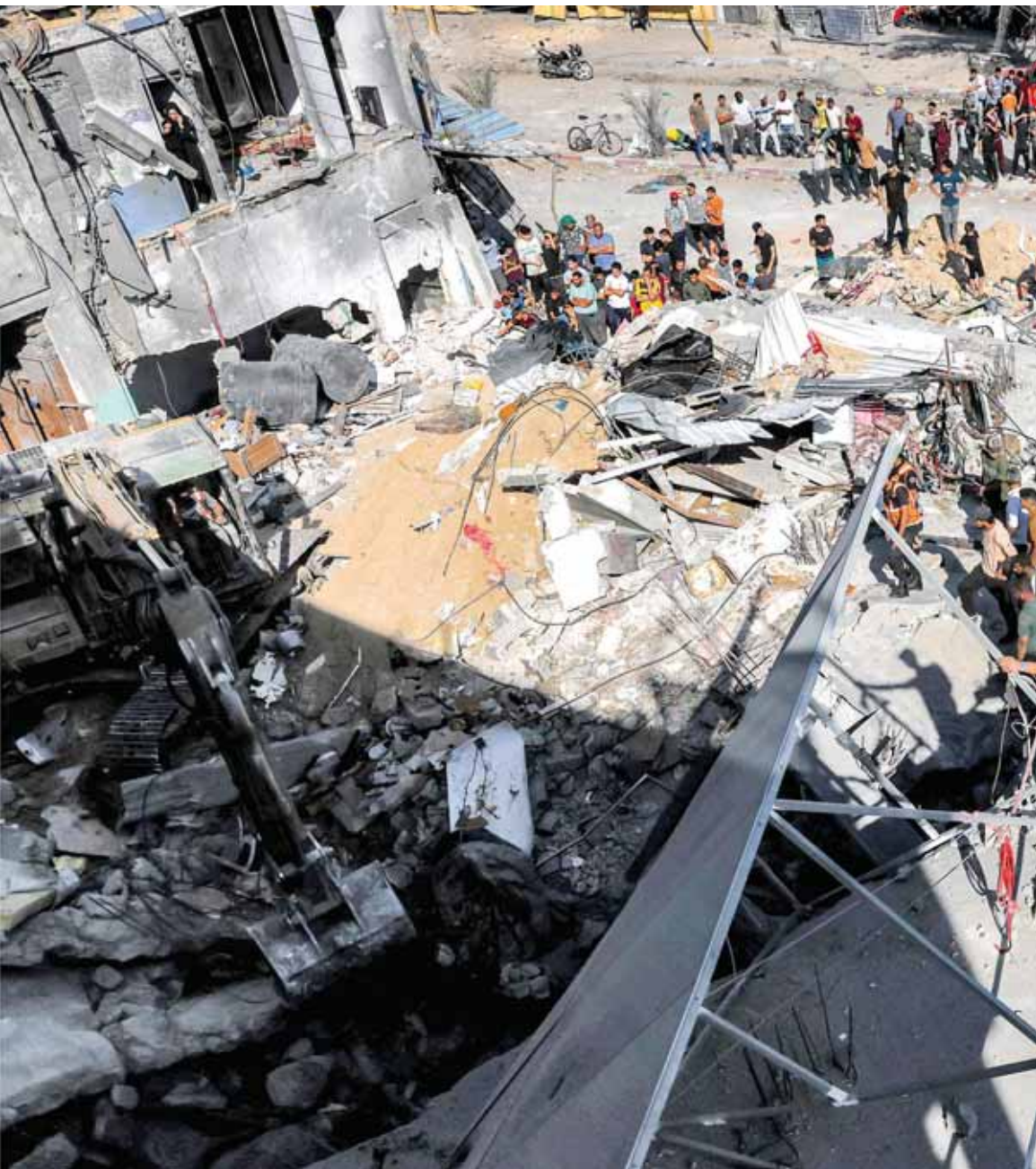
People stand by as civil defence workers search for victims and survivors in the rubble of a building that was hit by Israel
