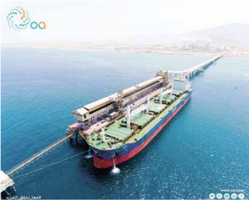
View of Omifco's jetty facilities at Qalhat near Sur.
