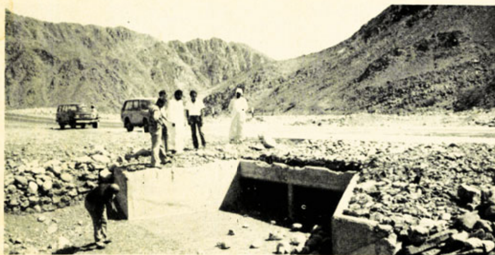
Inspection at a road worksite in the Interior.
