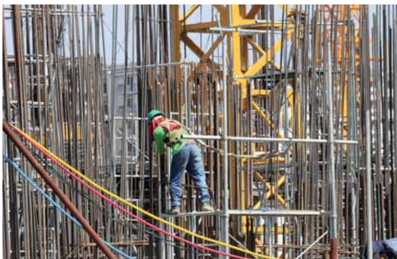
A worker installs steel rods at a construction site in Manila, Philippines. — Reuters
