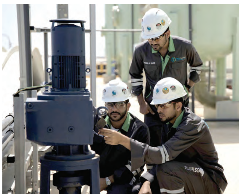
The plant demonstrated its ability to meet the total contracted water capacity of 105,000 metres 3 per day, marking a pivotal milestone for the project.
