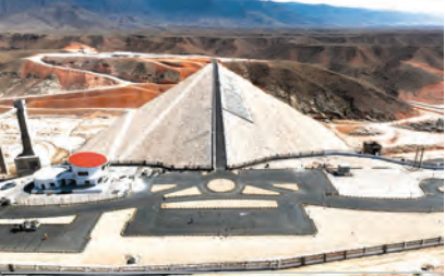
The dam boasts an integrated monitoring system. — ONA
