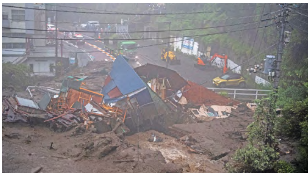
Debris at the site of a landslide following days of heavy rain, in Atami in Shizuoka Prefecture on Saturday (AFP)
