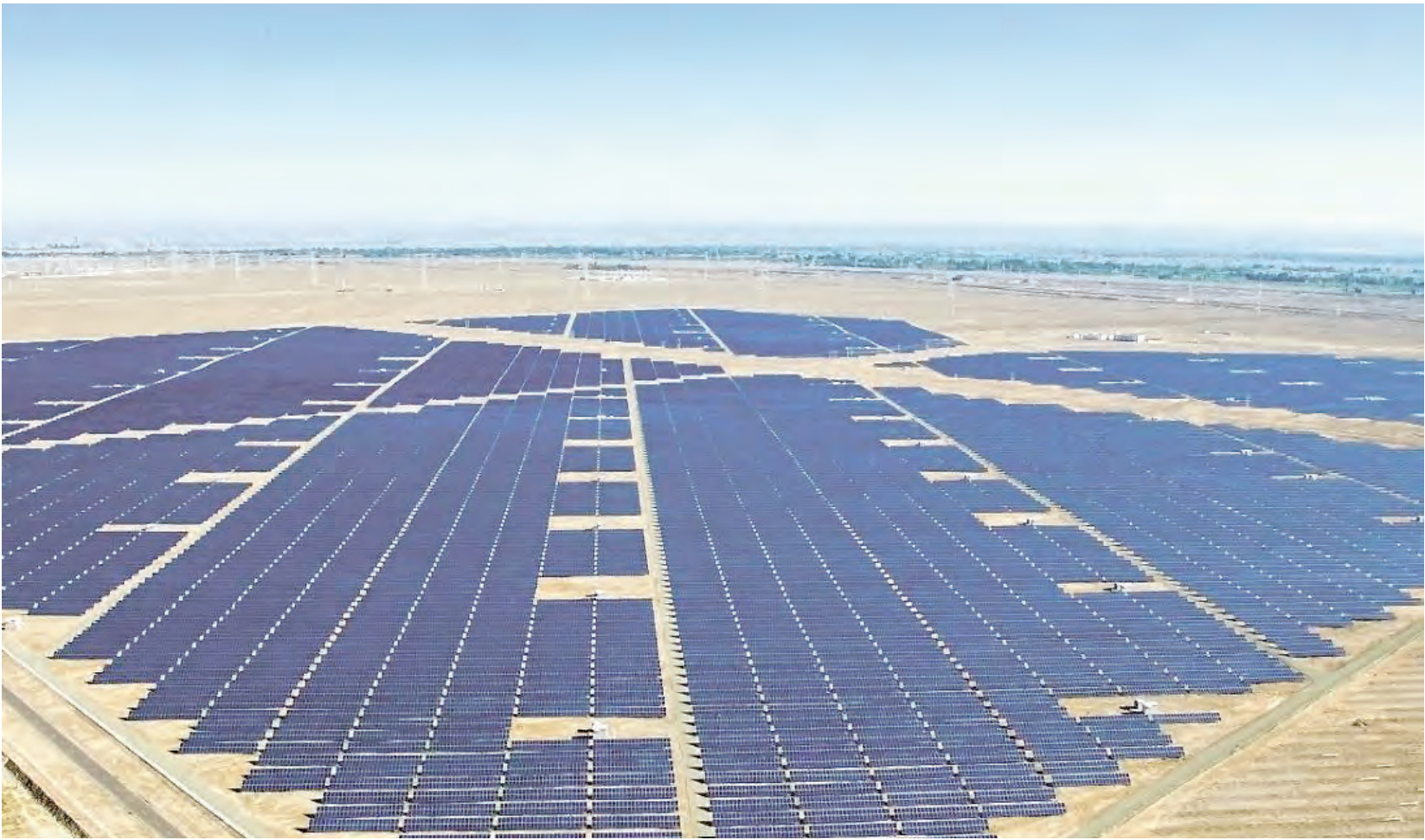
By 2023, Oman's commitment to renewable energy initiatives has gained significant traction, exemplified by the Dhofar Wind Power Project and the Ibri II solar project (pictured), which signify substantial progress towards achieving 30% renewable electricity by 2030.
