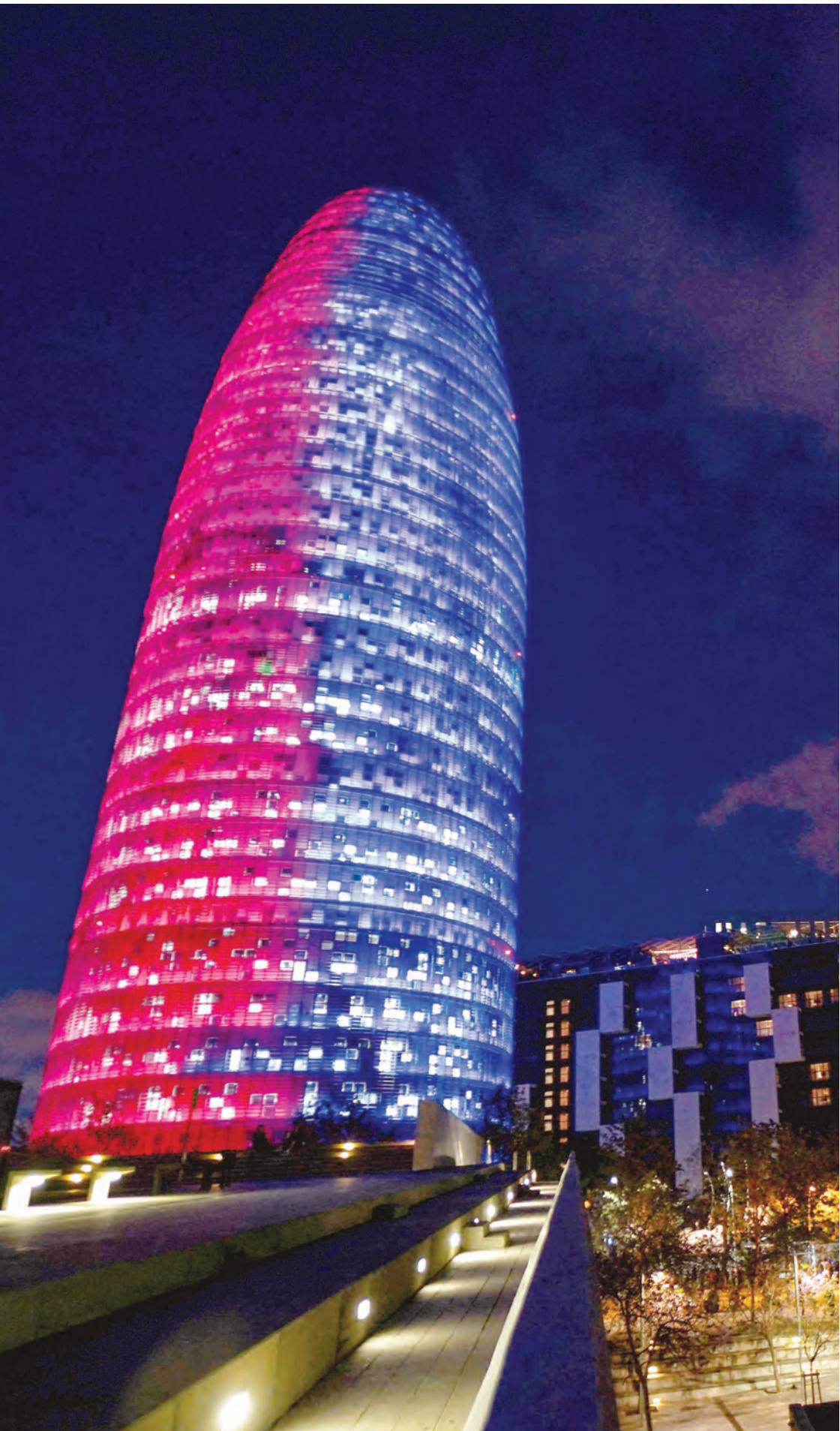
The picture shows a general view of French architect Jean Nouvel's building Torre Glories at night, in Barcelona. Recently, Glories Tower has become a member of the World Federation of Great Towers. – AFP
