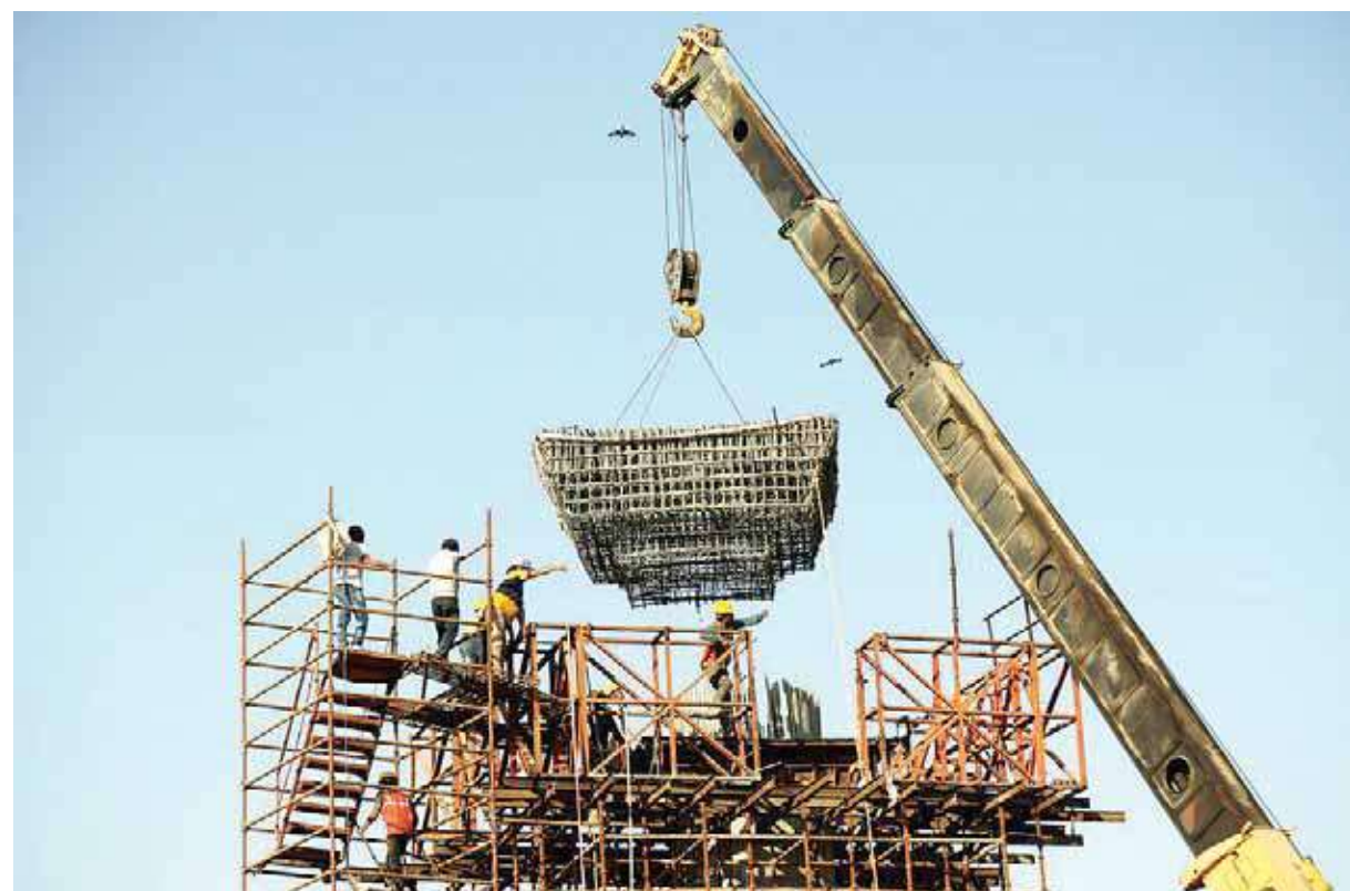
Workers build a pillar at the site of the metro railway flyover under construction in Ahmedabad, India. — Reuters
