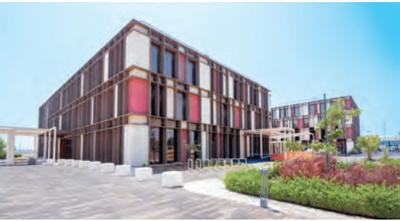
The Business Park brings a new workplace destination to the heart of one of Oman’s most established integrated communities.
