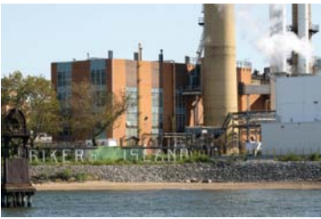
Rikers Island jail complex, seen from the Bronx borough of New York.
