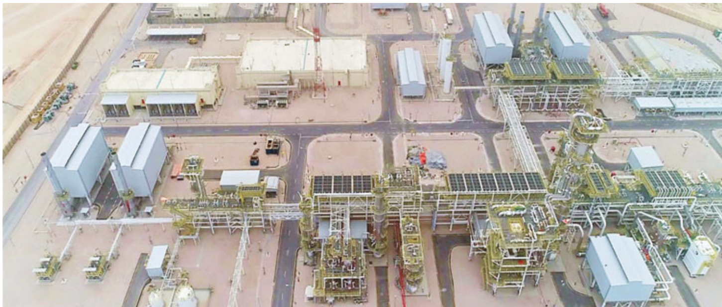
VITAL PROJECT: This vital project works on processing natural gas liquids extracted from gas networks into LPG. The plant is designed and built to the highest technical and safety standards. - ONA
