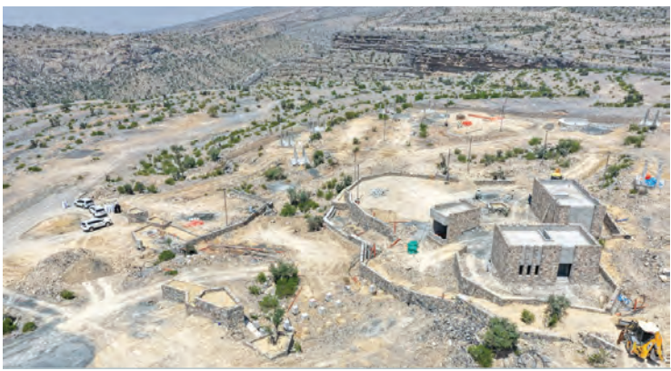
The Misfat Al Abriyeen rehabilitation and development project is 40 per cent complete.
