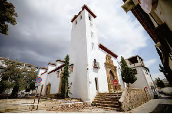
Spain’s cherished tourist hotspot of Granada was in shock on Saturday after a rare 5.0-magnitude earthquake woke residents in the middle of the night and damaged buildings. But officials confirmed no casualties or serious damage, notably to the southern city’s Alhambra palace, a Unesco-listed jewel of medieval Islamic architecture. The tremor took place shortly after 1:00 am with its epicentre in the town of Alhendin. — AFP
