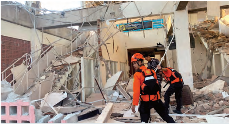
Rescuers inspect a heavily damaged building after an earthquake in Sikka, Maumere, Indonesia. — Reuters
