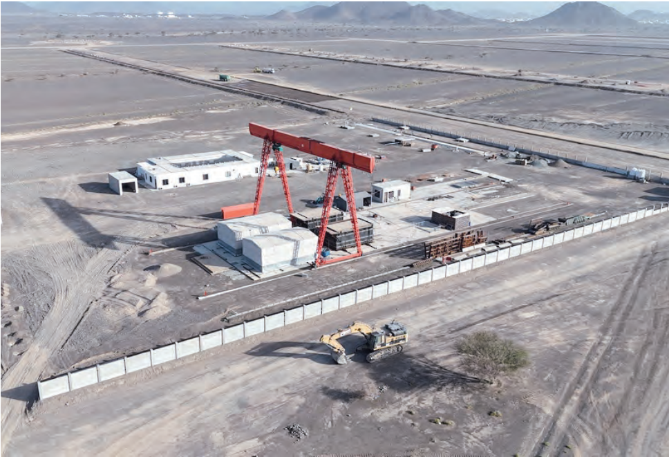
The city has begun infrastructure works covering 1.34 million square metres of its planned 9 million square metre site.
