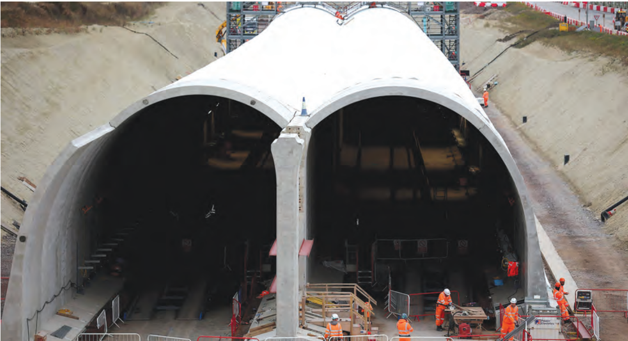
Construction workers work at a construction site near Wendover, Britain. — Reuters
