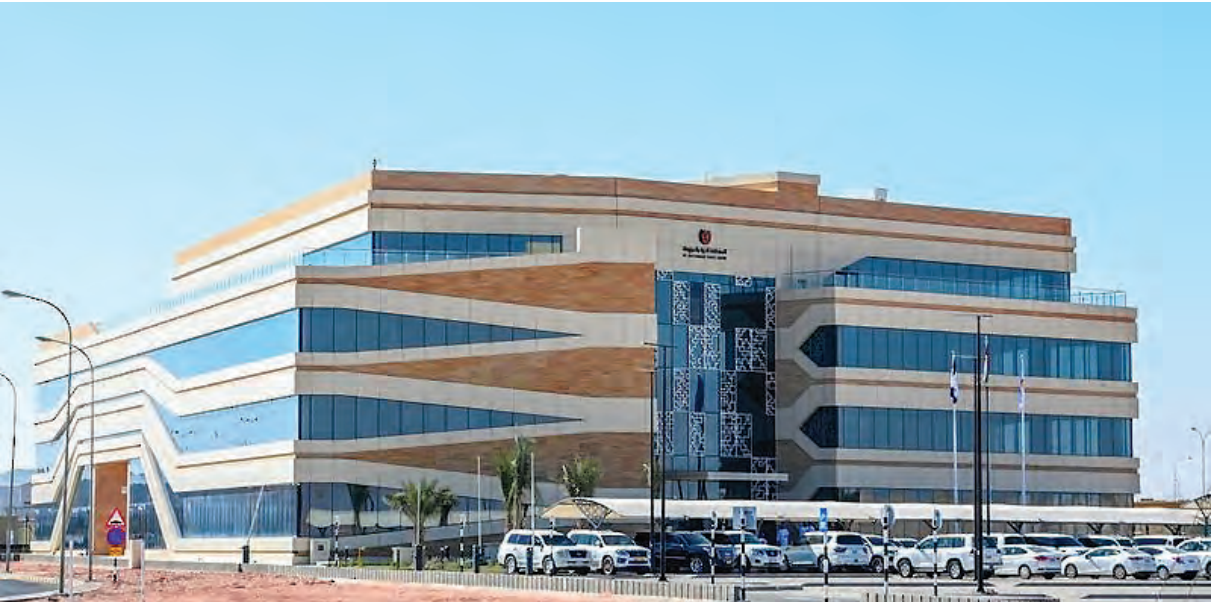
Al Mazunah Free Zone is an important hub straddling Oman's border with Yemen in the south
