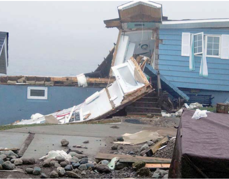
A view shows a damaged home in the aftermath of Hurricane Fiona in Port Aux Basques, Newfoundland, Canada. — Reuters
