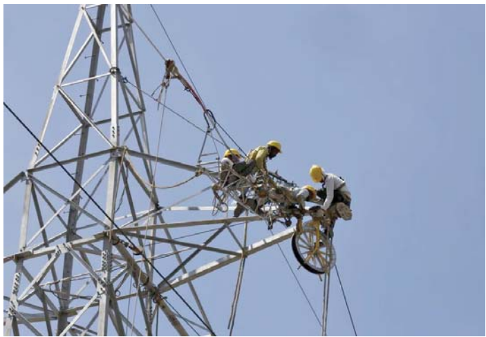
Workers of Torrent Power Limited install cables on electric pylon on the outskirts Ahmedabad, India. — Reuters
