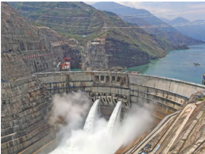
This aerial photo shows the 289m tall Baihetan Hydropower Station in Zhaotong, in China's southwestern Yunnan province (AFP)
