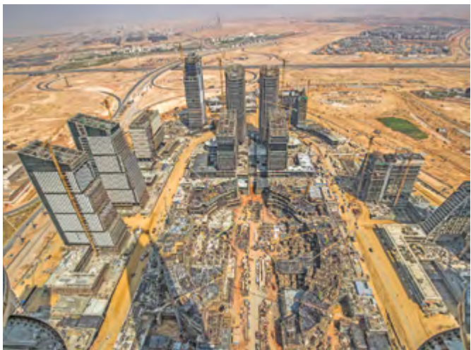
This file photo shows construction work at the business and finance district of Egypt’s ‘New Administrative Capital’ megaproject (AFP)
