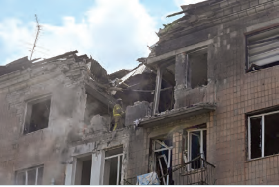
Rescuers search the rubbles of a damaged residential building in Kharkiv. — AFP
