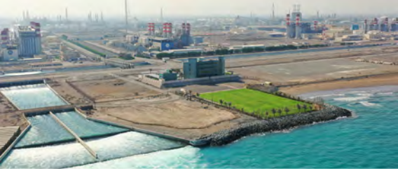
Majis specialises in industrial water solutions and utilities serving Suhar’s industrial sector.
