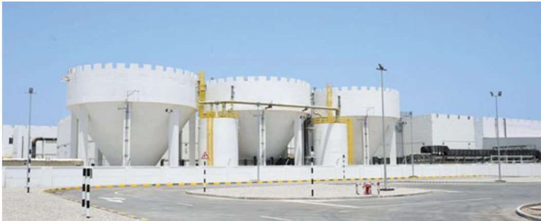
The maintenance work is expected to continue for 72 hours from 6am on Thursday to Saturday (March 11, 2021). — OMA
