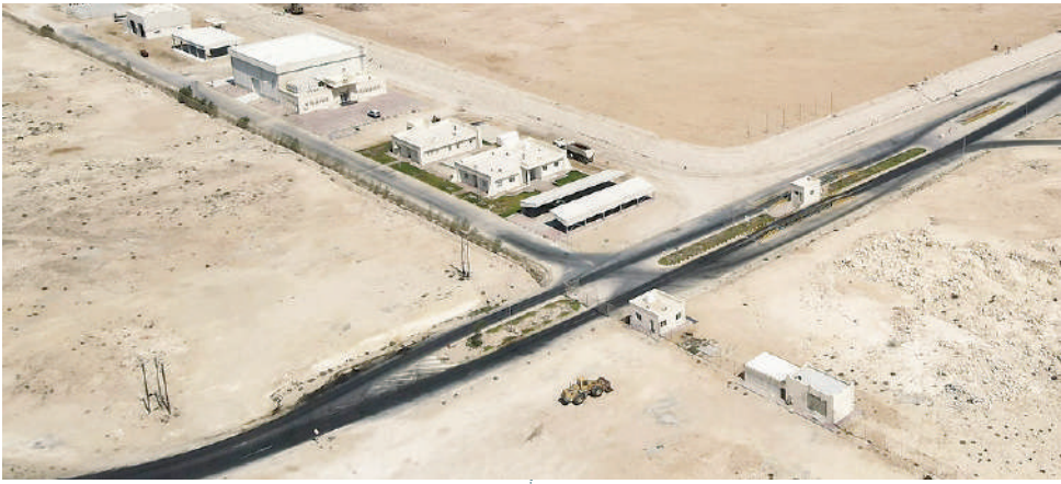
be’ah is building an integrated leachate treatment plant to process liquid waste generated from landfill decomposition.
