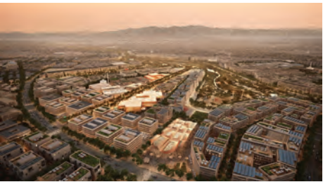
Sultan Haitham City has achieved full completion of land preparation and levelling works, while progress continues on main roads, underpasses, utility networks and bridges.
