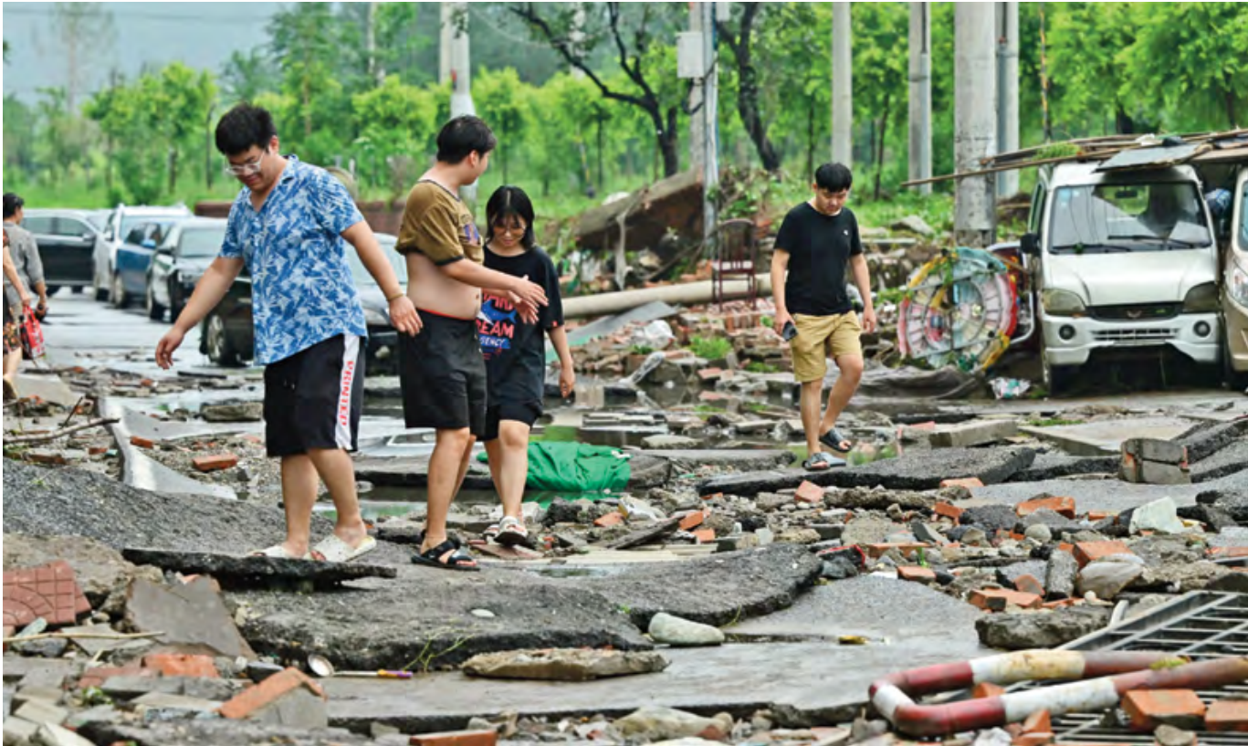
People inspect a damaged road following heavy rains in Fangshan district in Beijing on Tuesday (AFP)
