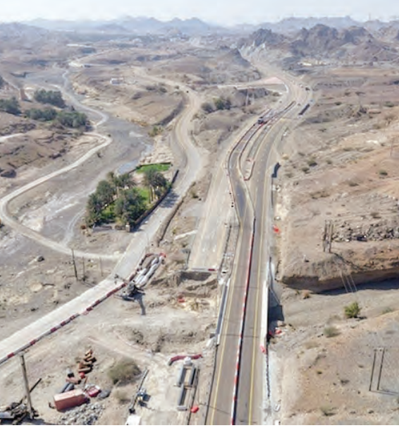
The construction is due to the road’s strategic importance in connecting border crossings.
