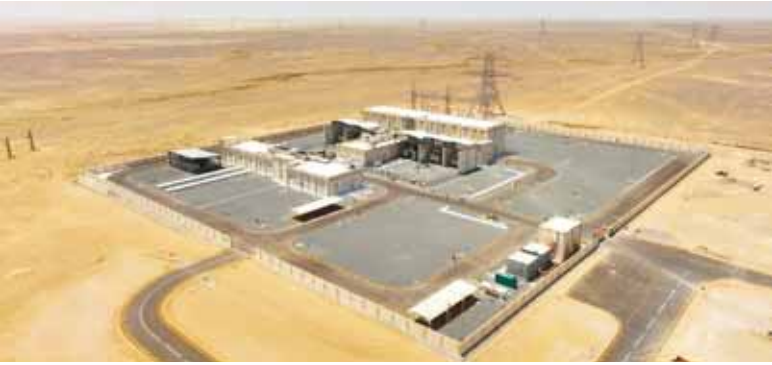
The project is one of the strategic and significant initiatives in the sector.
