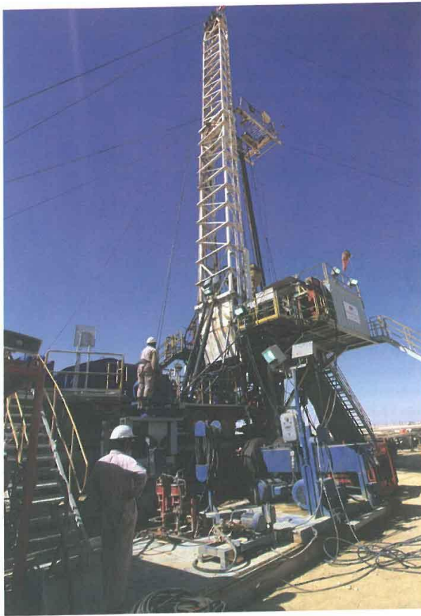
Ongoing maintenance at an oil rig
